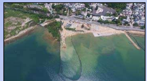
Silt curtain at Lung Mei Beach, May 2018
