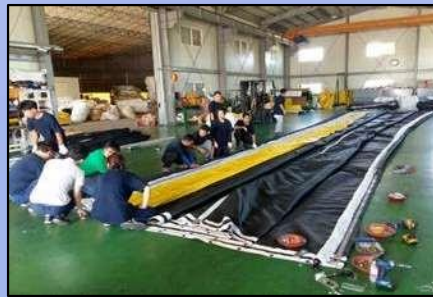
Fabrication of silt curtain
