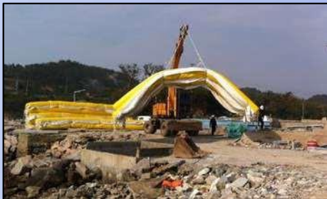
Handling of the silt curtain
