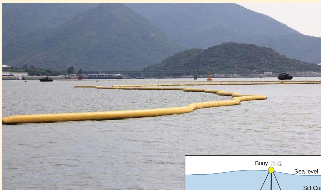
淤泥屏障 Silt curtains
