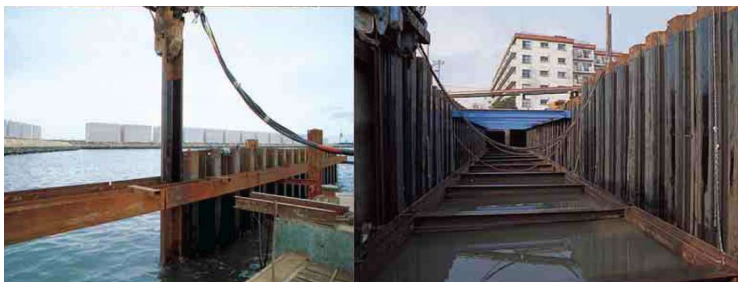
Installation/Extraction of Sheet Pile by Vibratory Method
